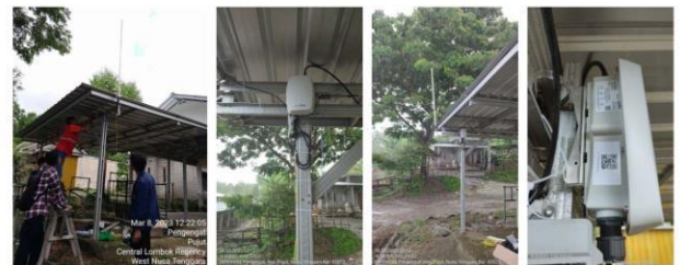
Gambar 3. installasi Gateway
